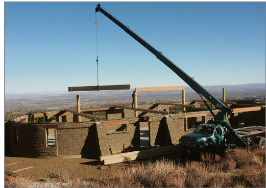
Figure 10. Truck crane placing ridge beam.
