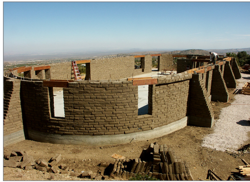
Figure 4. Round end and buttresses.
