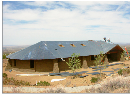
Figure 12. Corten steel roof.
