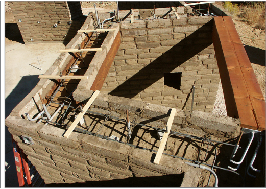
Figure 8. Bond beam on top of the wall at entry.
