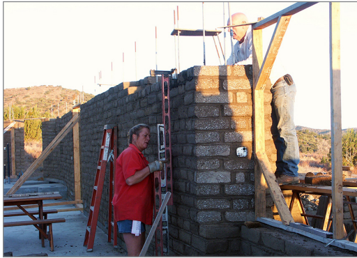
Figure 7. Using the vertical level.
