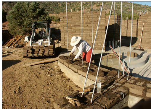
Figure 6. Laying block around the steel rods.
