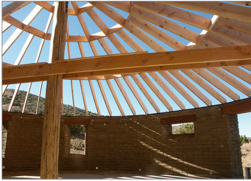
Figure 11. Rafters at west end .
