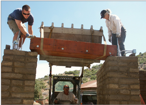
Figure 9. Setting the front door header.
