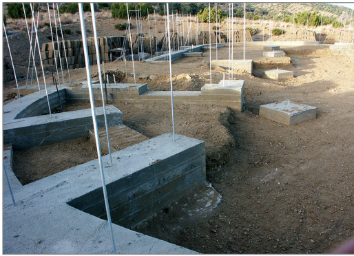
Figure 3. Galvanized steel rods.
