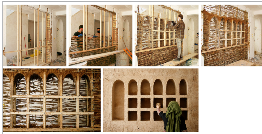
Figure 2. The building process of the earth wall partition and final plaster.
