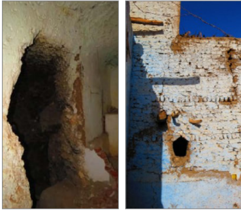
Figure 6. Holes present in the wall (left) 'Bab El Hagar' (right), Source: Mahmoud R. 2016.
